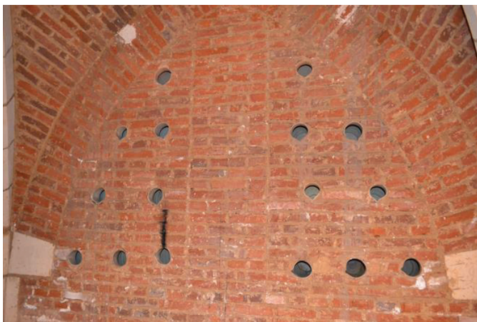
Figure 1: An example of the acoustical pots in the phonocamptic cave at Noyon.
